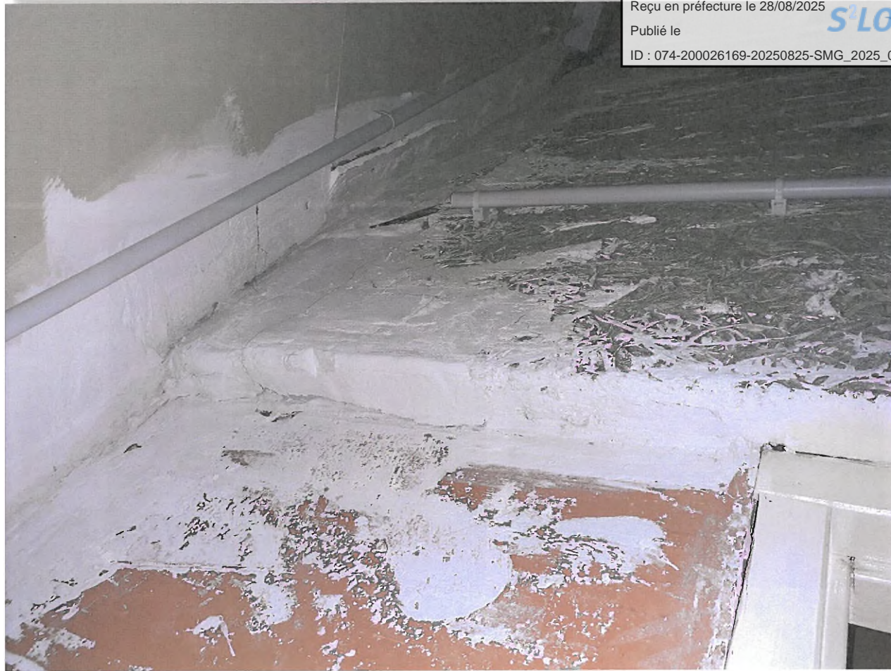
Fissure cloison combles 2022
